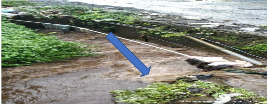
Plate 2: Water diverting from the Main drainage channel at Buea Town Neighbourhood
