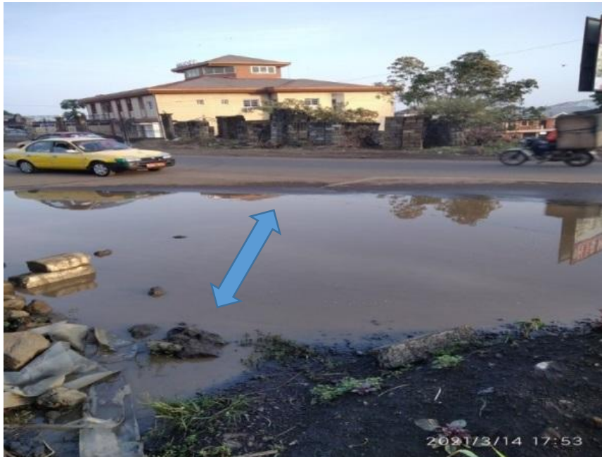
Plate 1: Lack of Drainage Infrastructure at Mile 17
